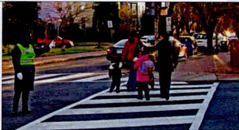
High-visibility crosswalks use parallel markings that motorists see more easily compared to traditional crosswalk markings.
